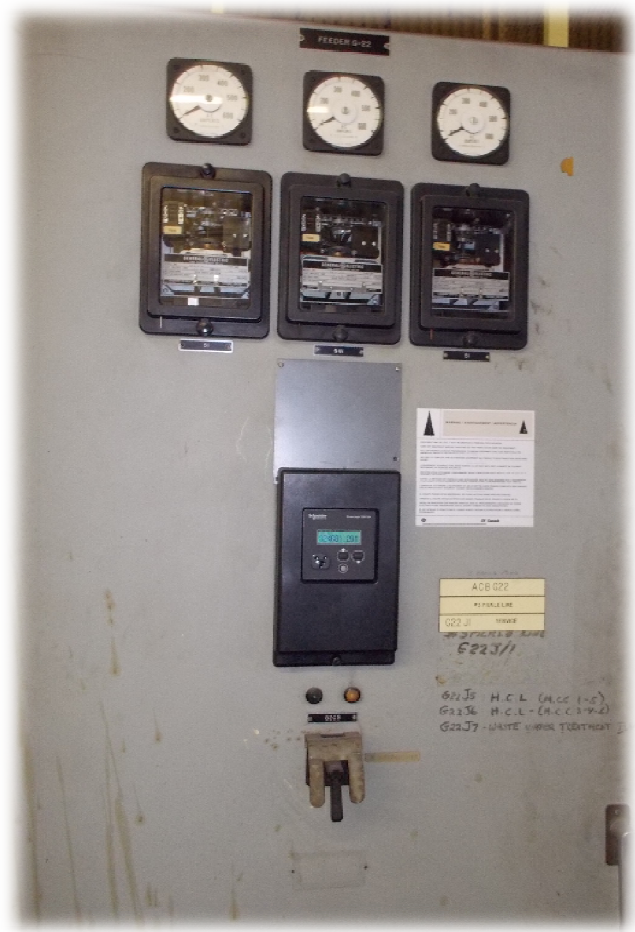
Analog Power Consumption Meter to Digital ION 7330 Meter
